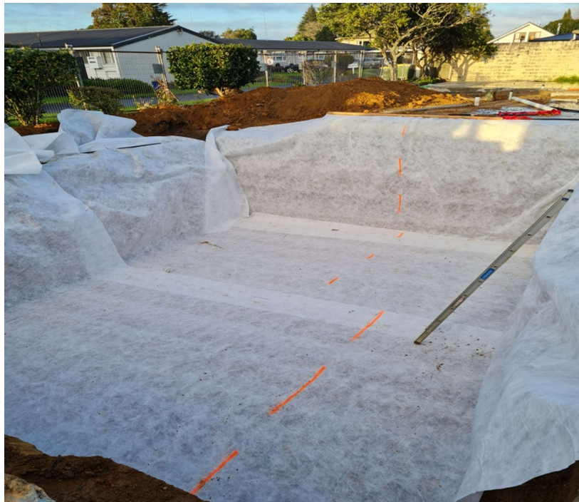
Geotextile Fabric Placement
