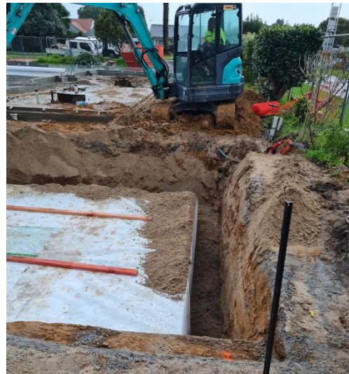
Wrapped StormCell Modules & Back-Filling
