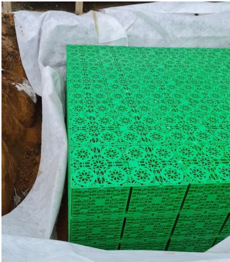
Completed StormCell System Construction
