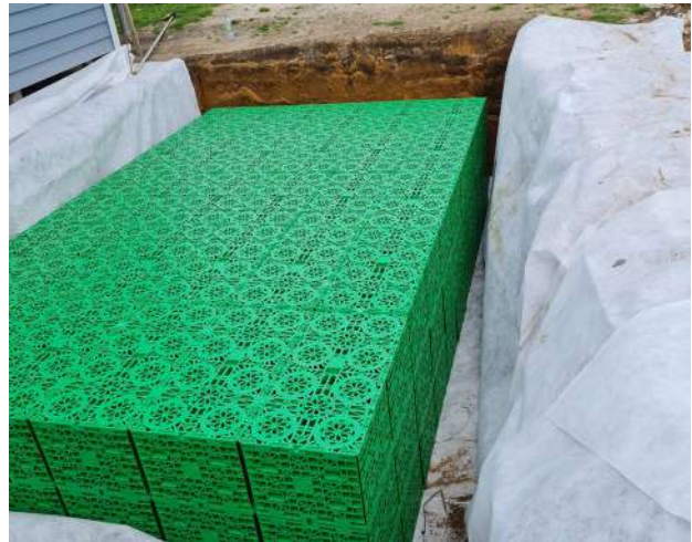
Wrapped StormCell Modules & Back-Filling
