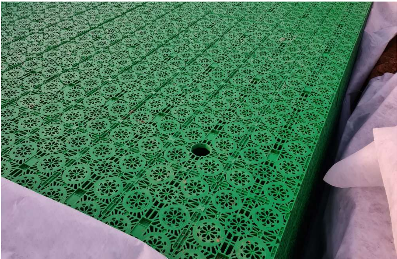
Completed StormCell System Construction
