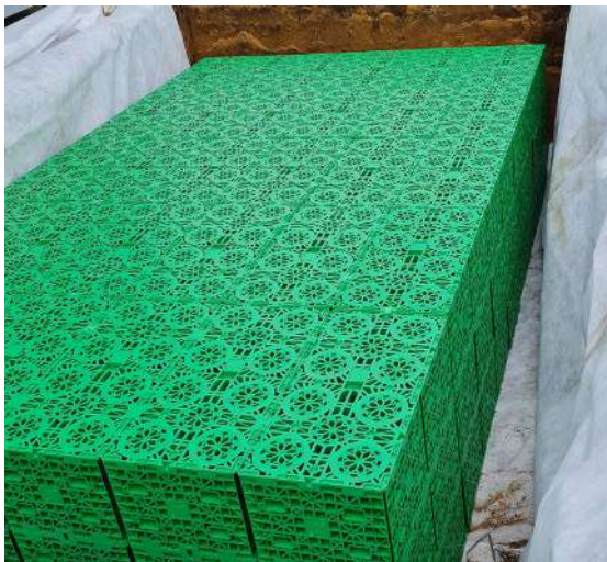
Completed Tank Construction
