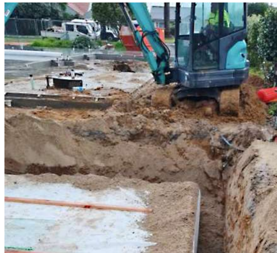
Wrapped Tanks & Back-Filling
