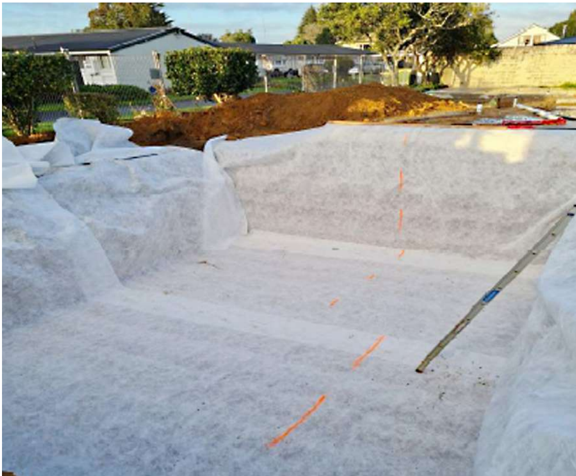
Geotextile Fabric Placement
